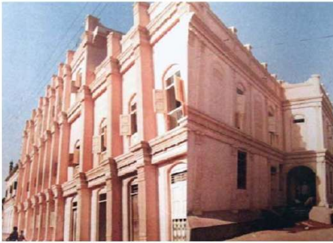
Facade of the restored Zakavi Haveli in Burhanpur where Syedna Zakiyuddin RA resided
