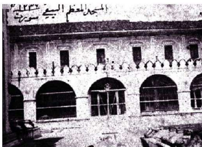
Masjide-Mo'azzam, a century before its restoration
