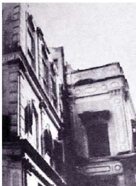
The old building of Darse-Saif
