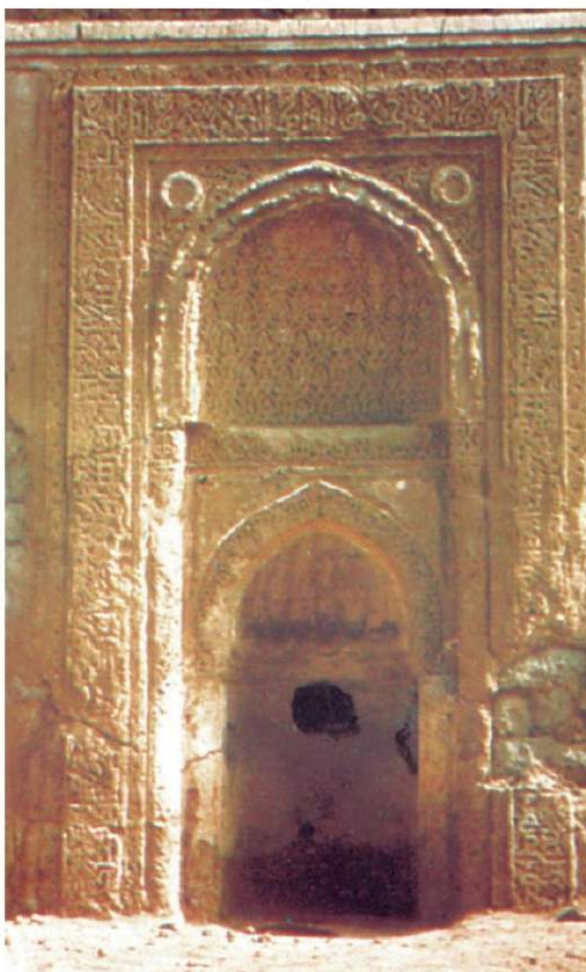
The mihrab of Syedna Zueb RA 's masjid before restoration
